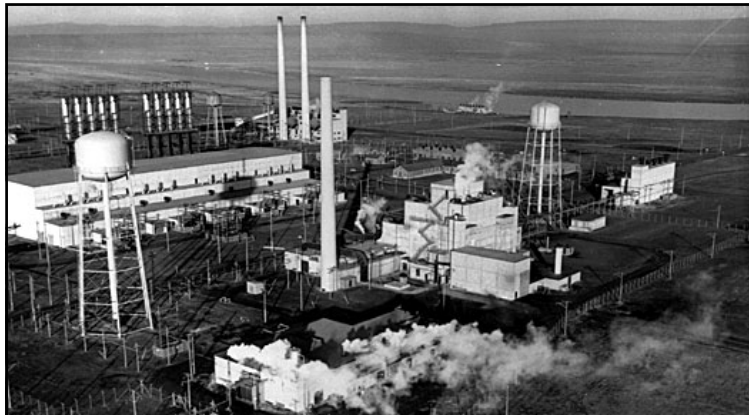
Hanford: Completed in September 1944, the 250,000 kilowatt B Reactor was the world's first large-scale plutonium production reactor. Two hundred tons of aluminum clad uranium slugs the size of rolls of quarters went into tubes. Cooling water from the Columbia River was pumped through tubes around the uranium slugs at 75,000 gallons per minute. This and all other US production reactors are shut down.
